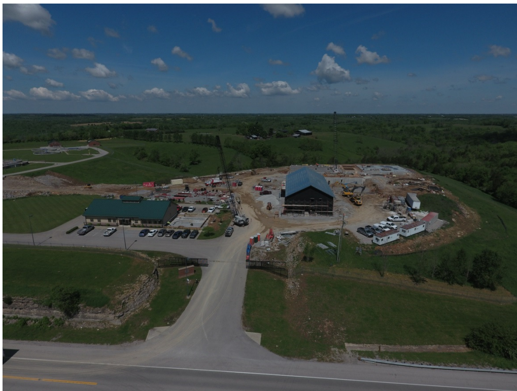
New Lower Howards Creek Water Treatment Plant Under Construction - May 2019
