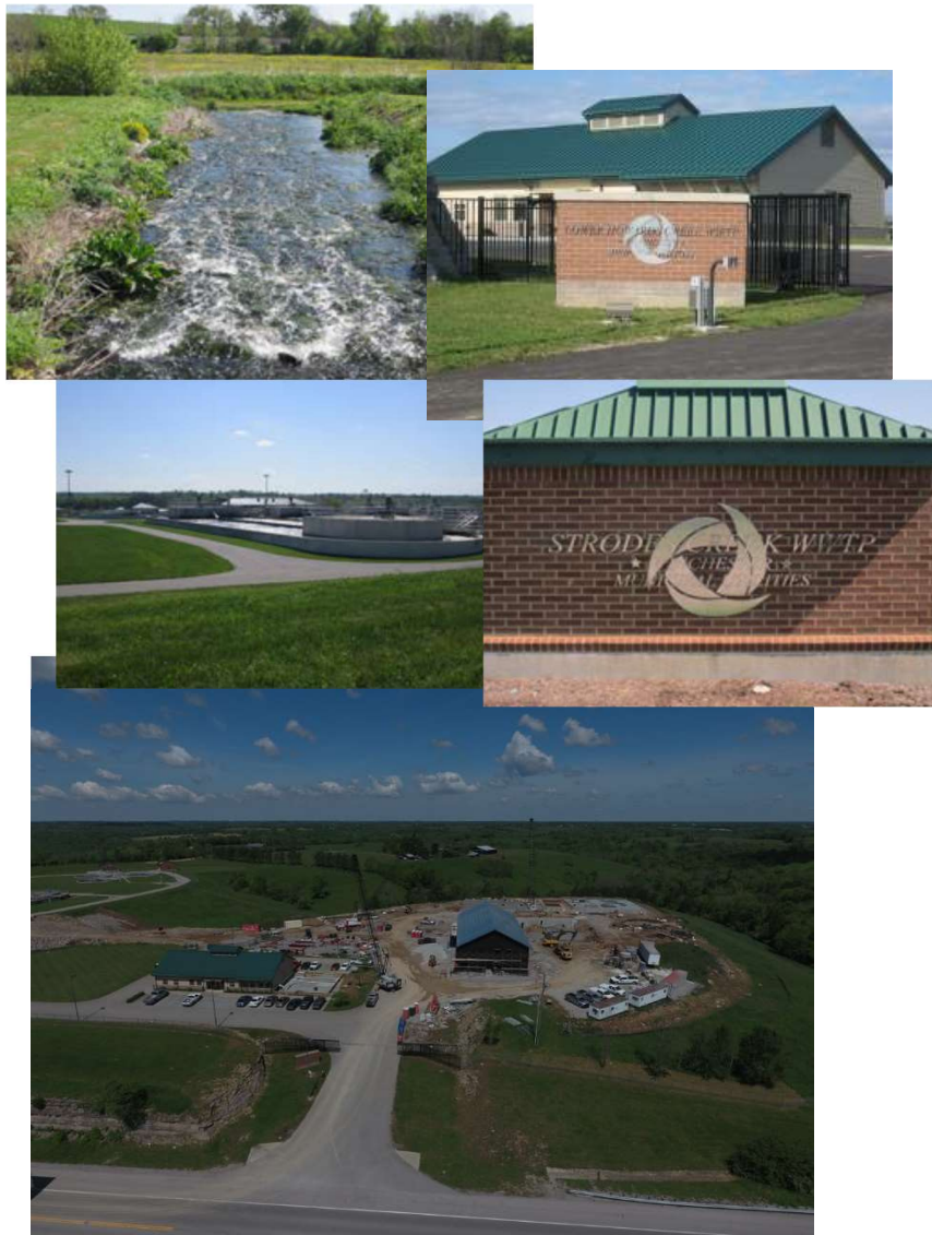
New Lower Howards Creek Water Treatment Plant Under Construction - May 2019
